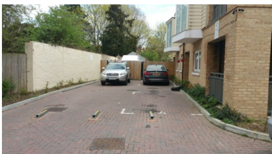
The parking for the main Flats. Only Two parking areas, and 3 bollard type parking protectors, add to the confusion. The constructed garage behind the wooden gates, that now demands a throughfare.
